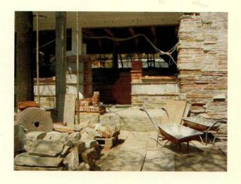
The support structure of the building is of reinforced concrete with walls of selected rocks, ceramic blocks and roman bricks.
